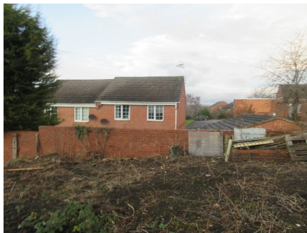
Photo taken from the application site facing north towards Nos 3 and 5 John Street
