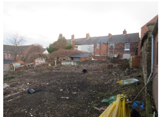
Photo taken from within site facing west towards the rear of buildings on High Street, showing site clearance
